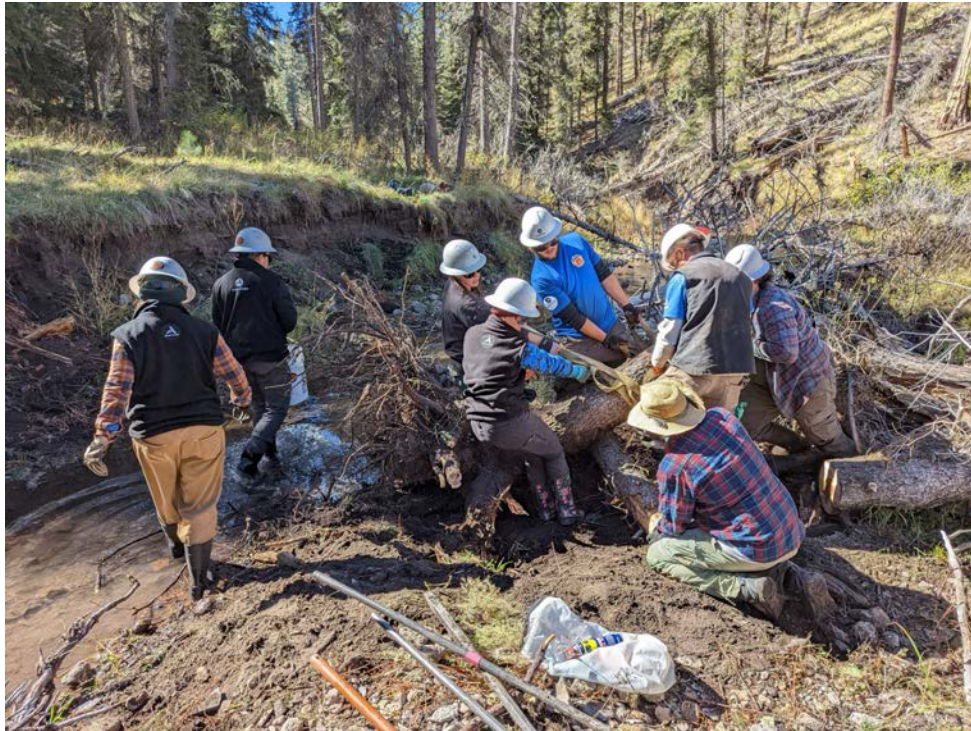
<= Installing Root Wad
