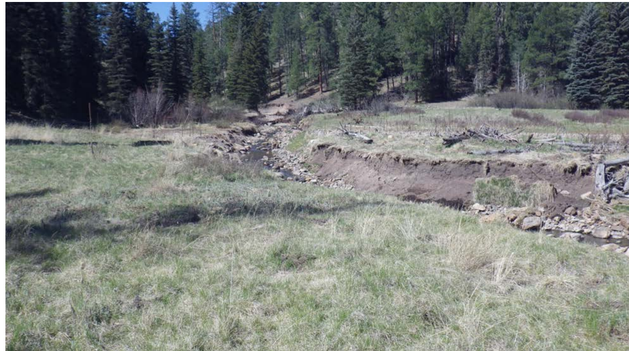
Significant Erosion and Sediment Loss 2017
